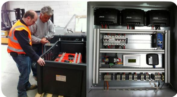
EnerSys Benelux built a complete 'off-grid' energy system for supply AC&DC uninterruptable power. Each system has 16 blocs Odyssey PC 1800 as back up. Charging of the batteries is done by 6 solar panels of 250Wp, supplied by our partner Soluxtec.
